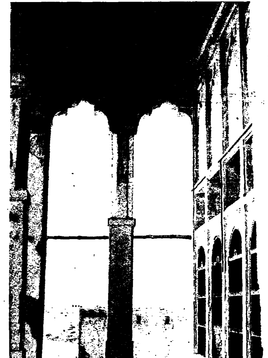
SITE: Sabhiya is the site of the desert palace of Sheikh Hamad al-Khalifa, the grandfather of the present ruler. The picture is the abandoned palace.
